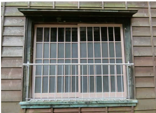
Fitting and repainting handrails ("Maruni Shoten" Kitchenware Store)
