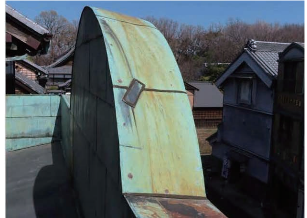
Copper plate joint caulking (House of Uemura)
