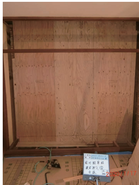
Installation of (structural plywood) bearing wall (House of Okawa in Den'enchofu)
