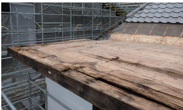
Before flat-roof repair (House of Koide)
