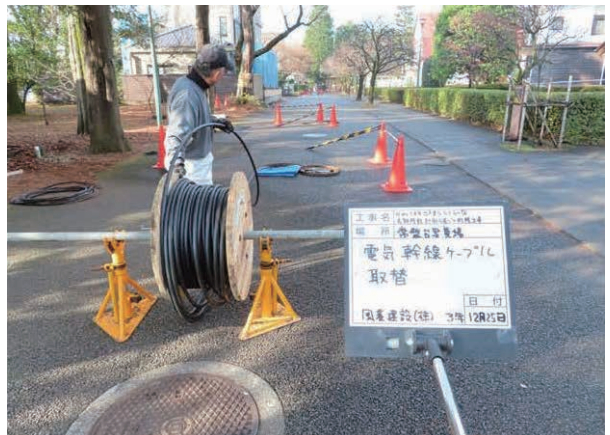
Electric trunk cable replacement (Tokiwadai Photo Studio)
