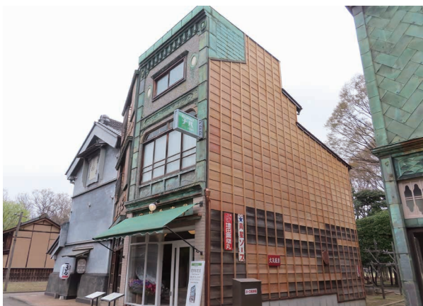
Exterior wall shitamita-bari (weatherboard) repair ("Hanaichi" Flower Shop)
