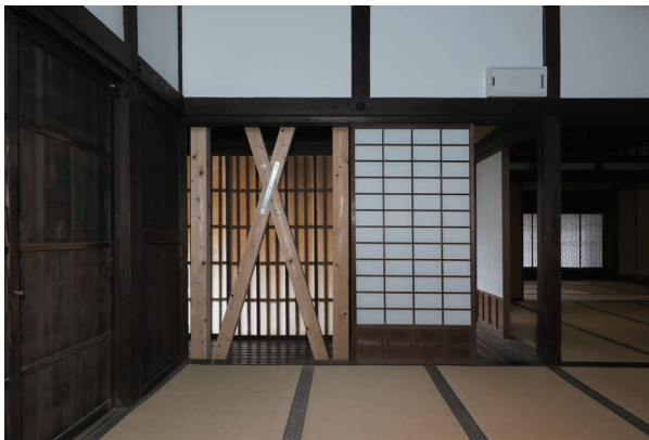
Installation of bearing wall (diagonal) (Farmhouse of the Tenmyo Family)
