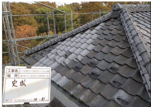
Tiled roof maintenance (Cosmetic Manufacturer “Murakami Seikado”)
