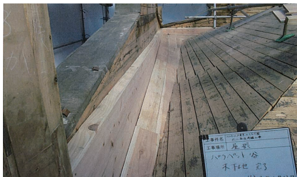
After changing the position of valley structure of the room (“Maruni Shoten” Kitchenware Store and Residence)
