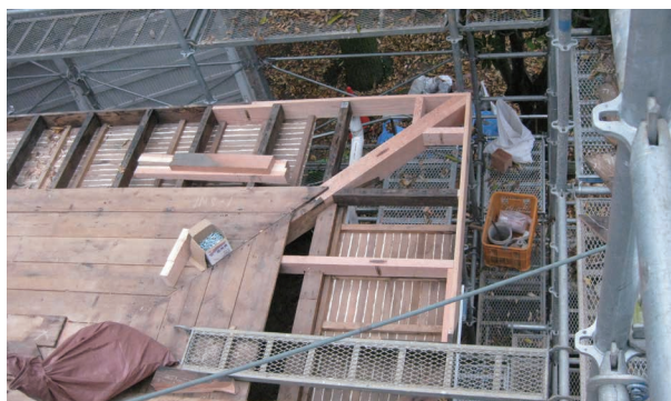
During flat-roof repair (House of Koide)
