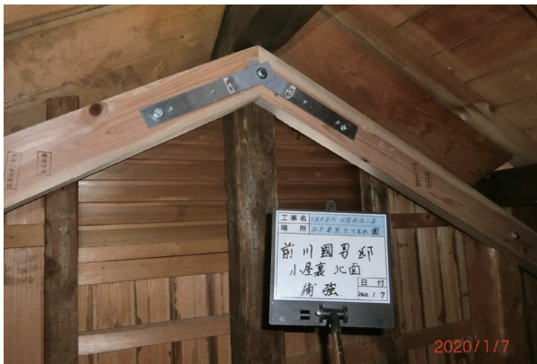
Installation of reinforcing material to roof frame (House of Kunio Mayekawa)
