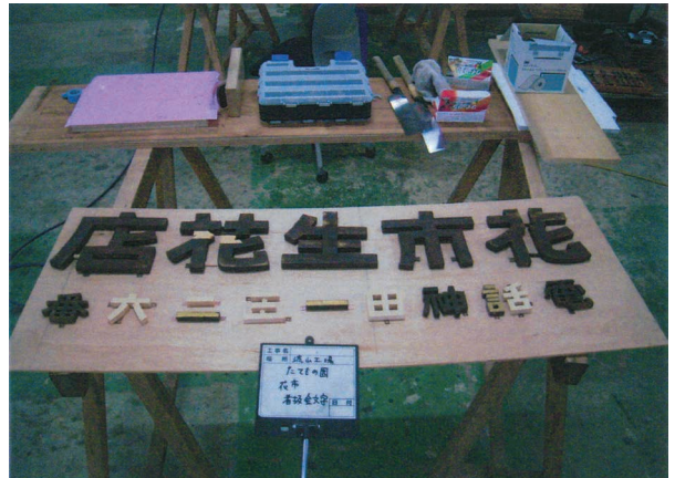
Signboard lettering repair ("Hanaichi" Flower Shop)
